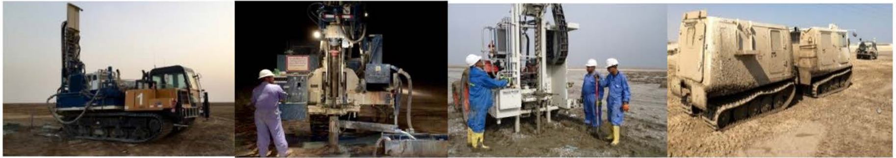
Figure 13. Special machinery deployed in field.
