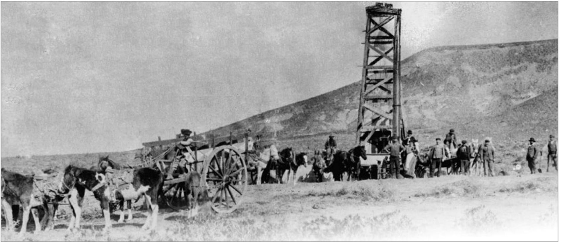
Figure 1. Drilling the early wells in Shell Diadema in the 1920s.
