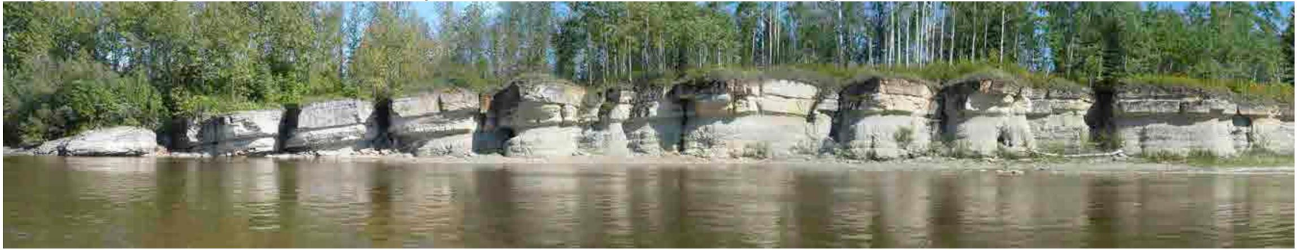
Figure 3. The northern limb of a 150+ metre fold at locality N88. Note the solution-enlarged joints in the outcrop. Unit 6 forms the 2.5 metre-thick resistant bed along the top of the outcrop.
