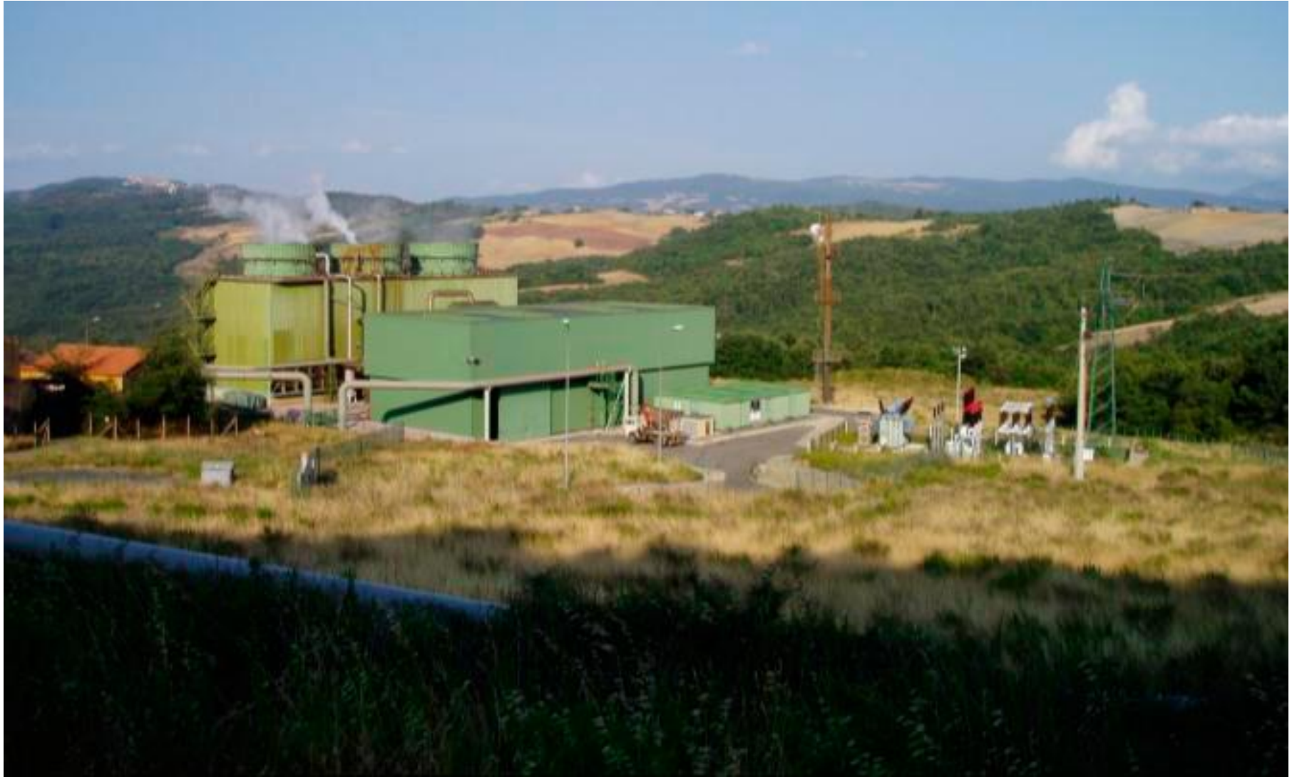
Figure 1. Larderello standard unit of 20MW dry steam electricity generating power plant – Italy (Source: SLR, unpublished, 2010).
