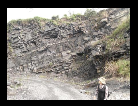
Joints and cracks distribute for network-shaped in 3D space.
