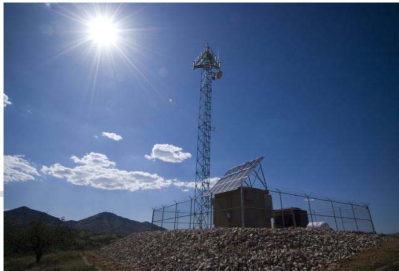
SBInet Tower in Border Patrol’s Tucson Sector (Courtesy of CBP)
