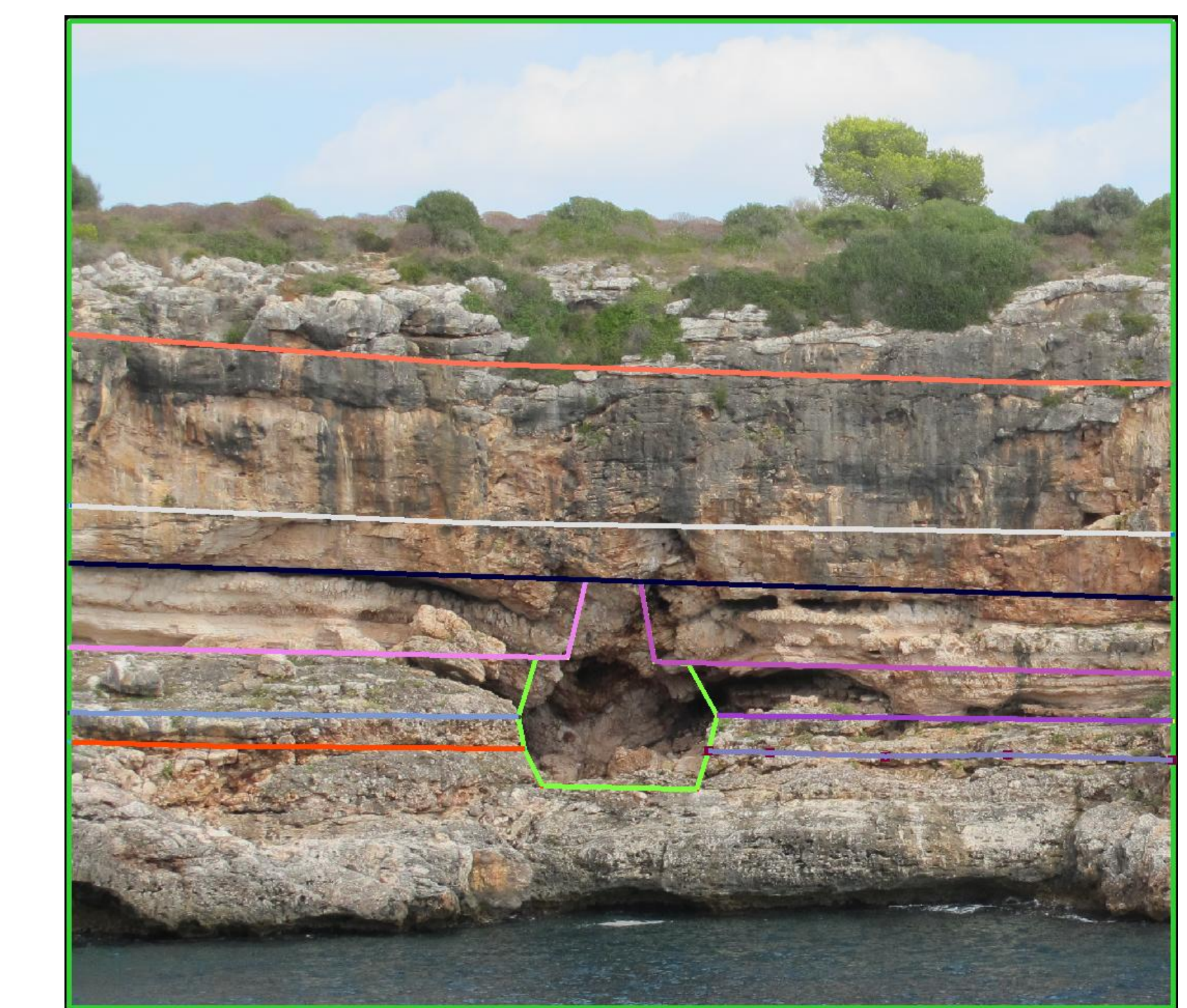
Fig. 10 – A simplified interpretation of the initial stage of the paleocave system for the purpose of the ELFEN computation. Only one cave that covers the main part of the system has been kept.
