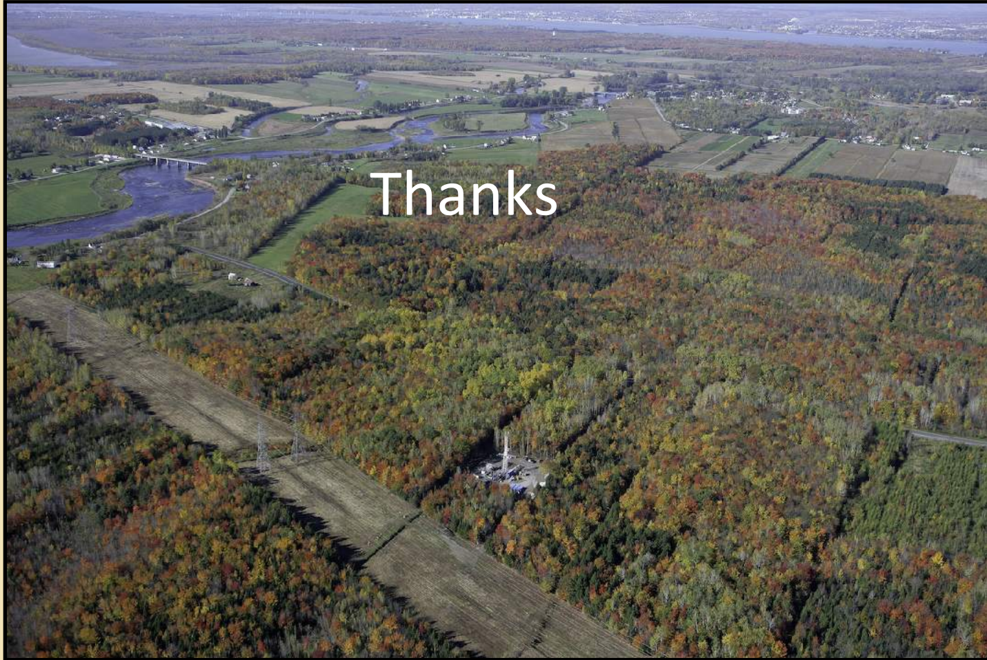
Foragaz Rig #2 drilling in Bécancour Area, Québec (September 2008)
