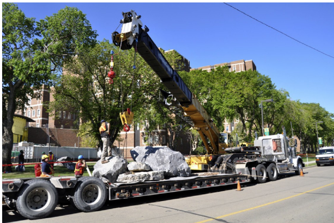
Figure 1: Installation in progress.
