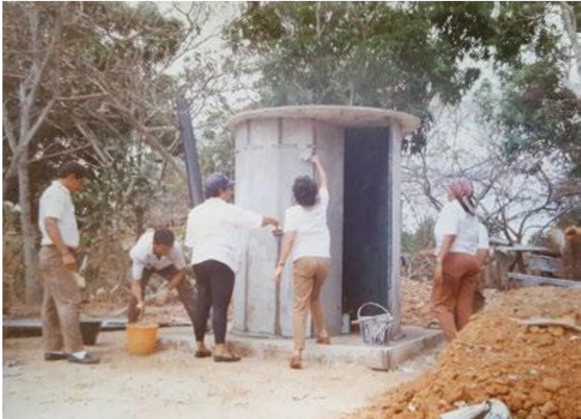
Figure 3. Community members helping to construct the VIP latrine under the direction of a Maraven technician.
