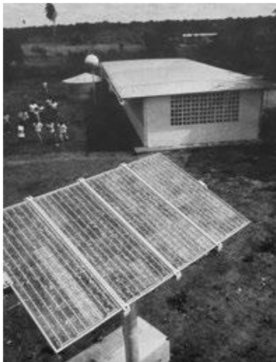
Figure 2. Model rural solar-powered school at El Manguito showing the slanted roof for rainwater collection, the gutter, and the tanks.
