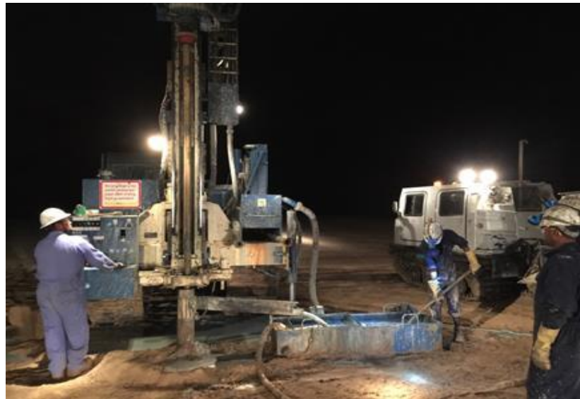
Figure 14. Pulling out in progress.
