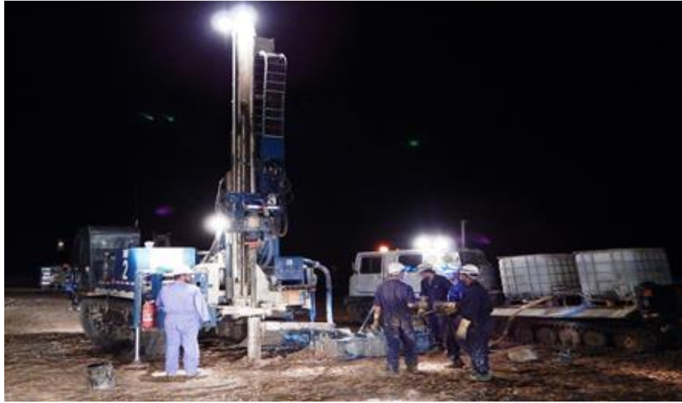
Figure 11. Night Shot-hole drilling in progress.
