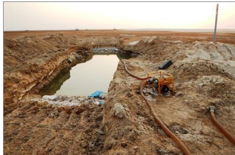
Figure 10. Pits for temporary storage of drilling water.
