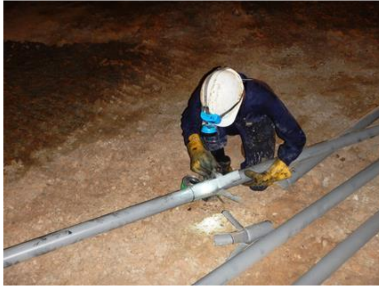
Figure 13. Casing being prepared.
