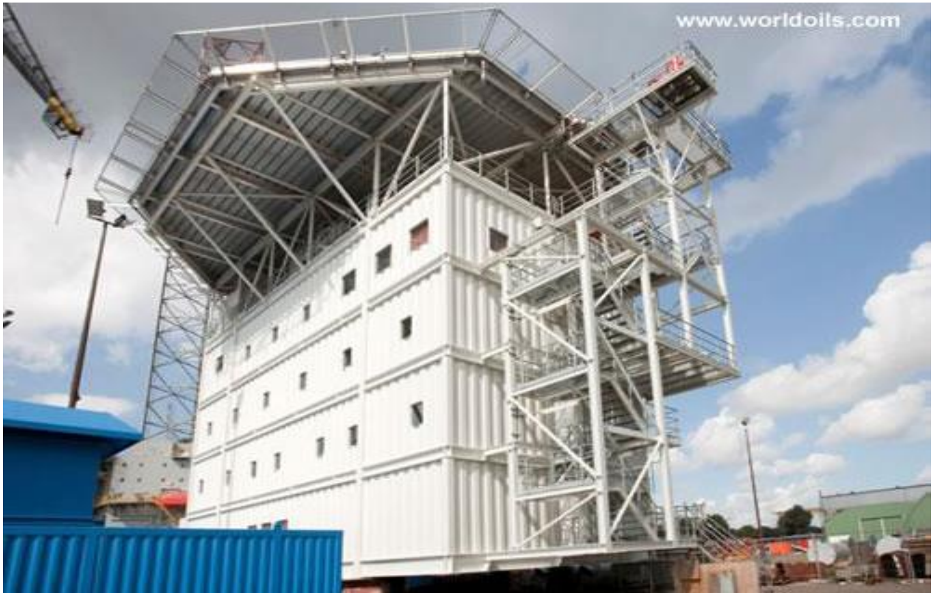
Figure 2. Offshore Rig Living Quarters Module (Macdonald, 2014).
