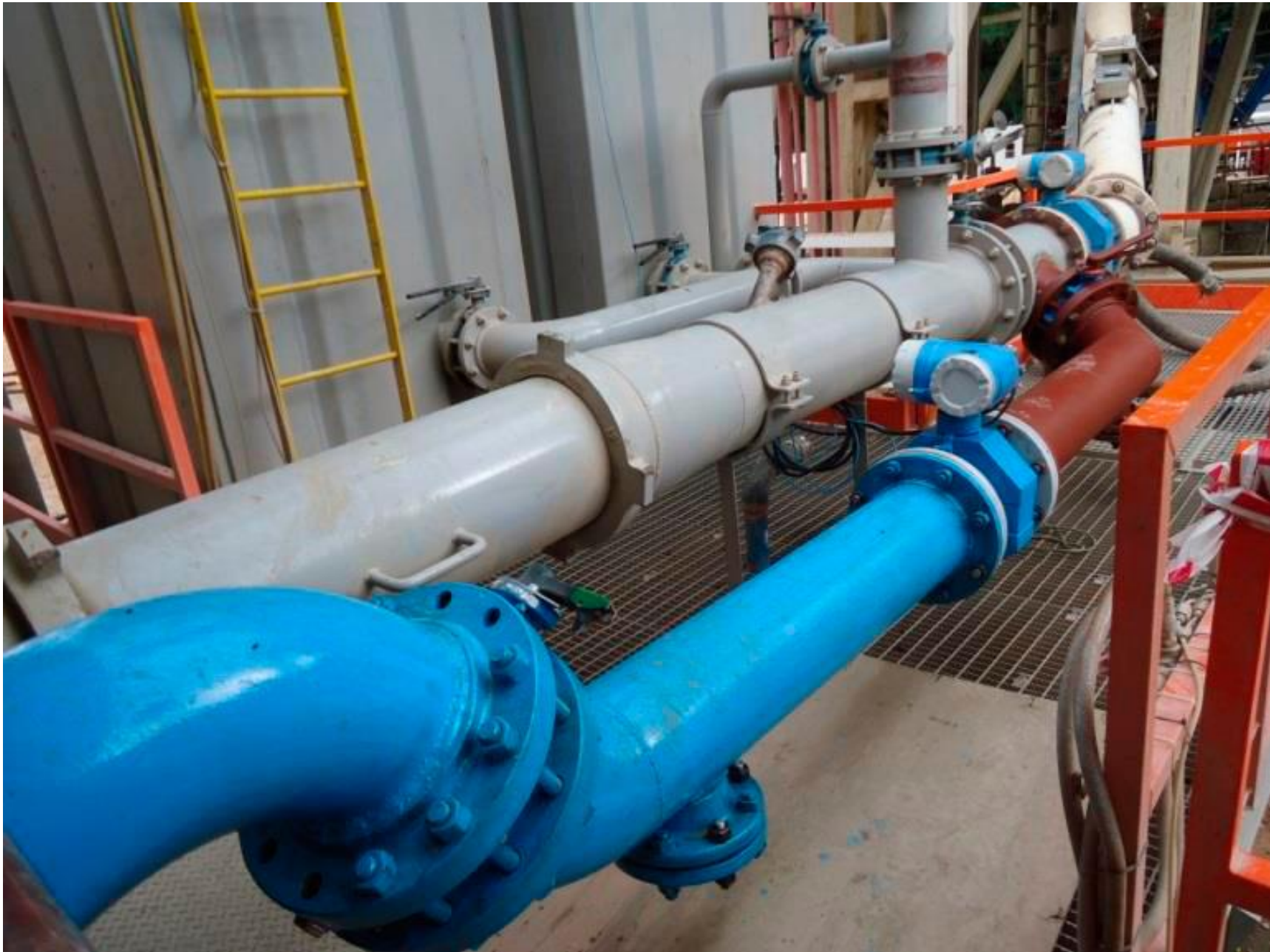
Figure 3. Electromagnetic flow meter.
