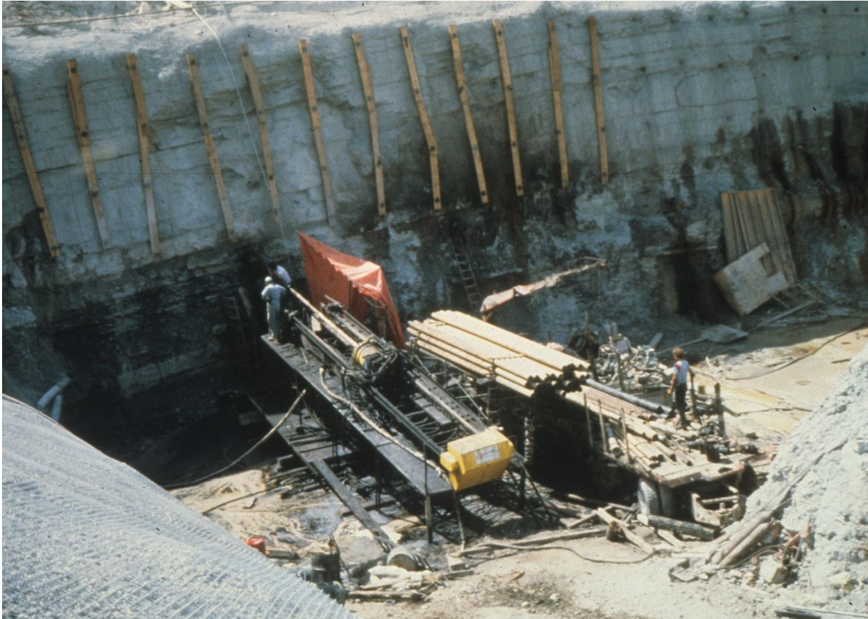
Figure 1: Hawker Siddeley Super Drill 150 in “The Pit”.
