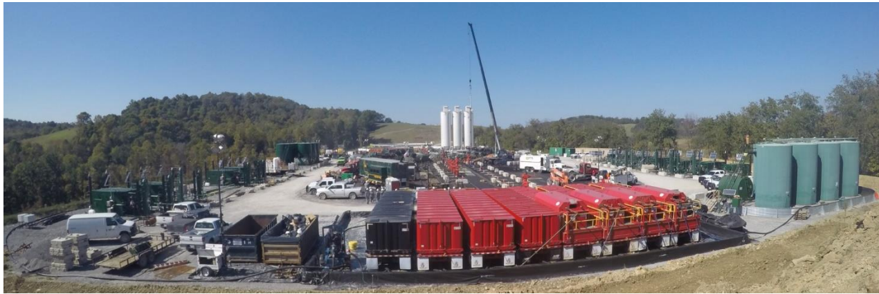
Marcellus well site with 50 multi-stage hydraulic fractured horizontal wells (Oct 2016)
