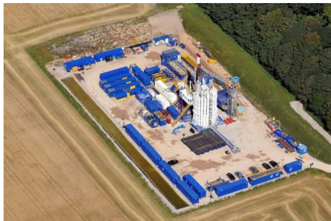
Well site at Weeton with Preese Hall hydraulically fractured (2011) vertical well targeting the Bowland Shale in Lancashire, England (abandoned & site restored, 2015)
