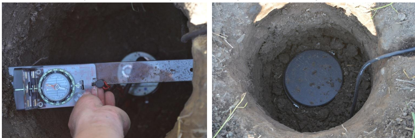
Figure 3: Shallow Posthole Installation
