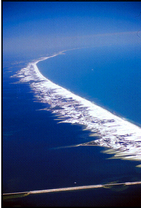
Figure 1. Expansive overwash deposits along the Florida Panhandle that occurred during Hurricane Opal (1995).
